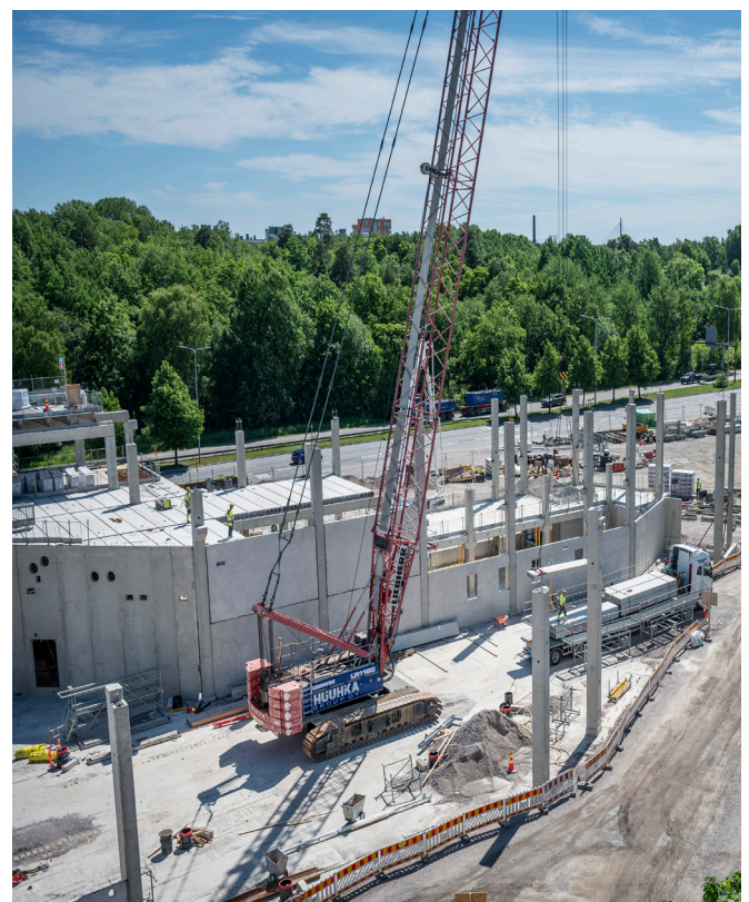
Overview of the Koskela depot construction site
