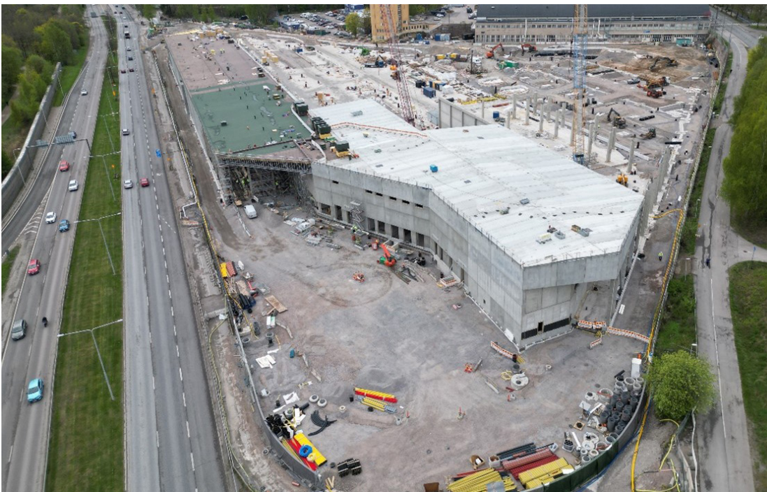
Overview of the Koskela depot construction site
