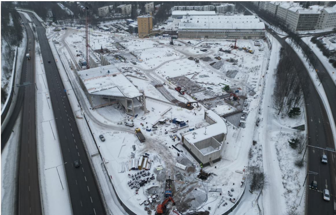
Photo: construction site on January 21, 2026
