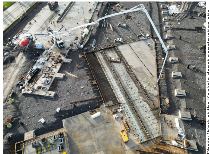
Photo: Work at the Koskela depot construction site
