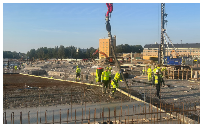
Photo 2: Concrete work at the construction site.
