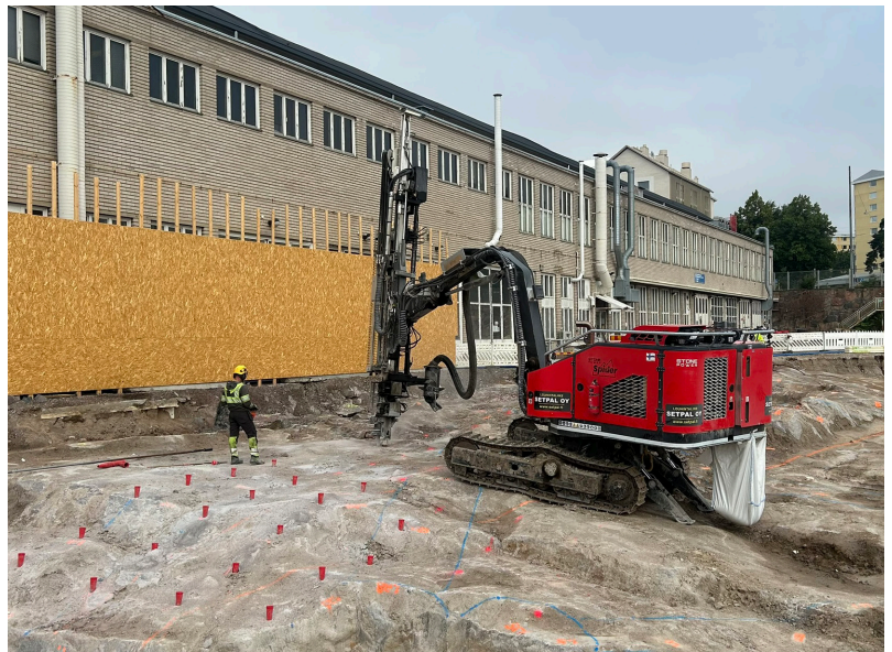
Photo: Drilling of the rock line for excavation.
